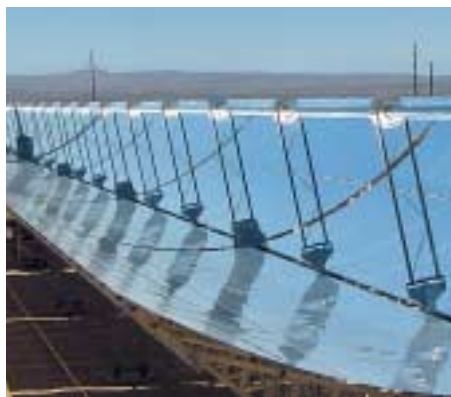
In the solar field, parabolic mirrors concentrate solar irradiation 80 times on an absorber tube.
