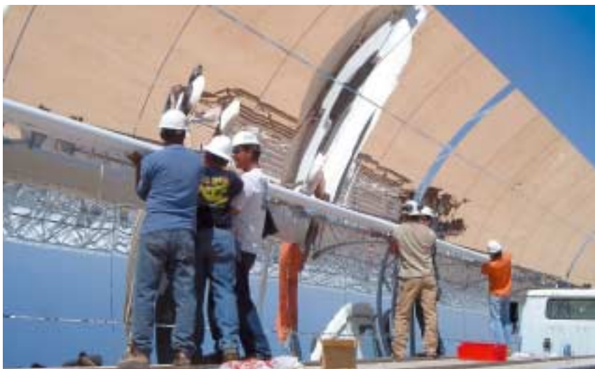
SCHOTT receivers being built into a mirror segment.
