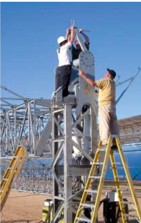
Construction of the drive pylon for a parabolic trough collector in California.
