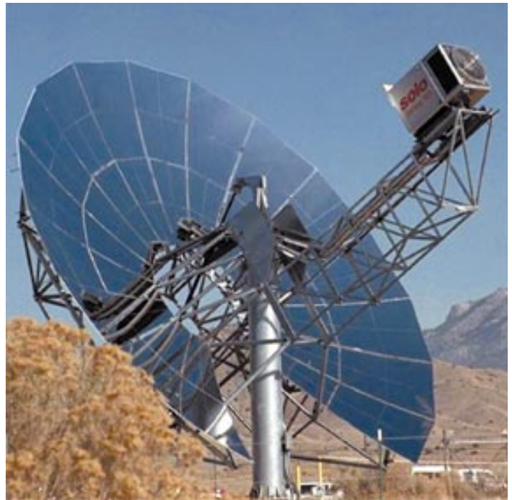
The Advanced Dish Development System is a 10 kW water pumping system developed by WG Associates for use by Native Americans in the southwest U. S.
