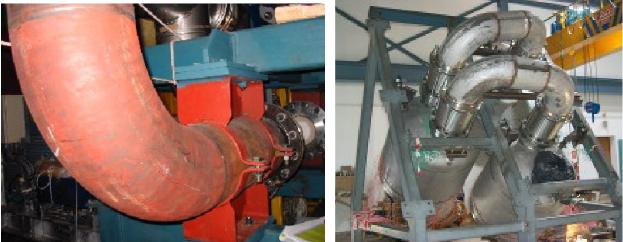
Fig. 11: Mounting of the gas pipes
