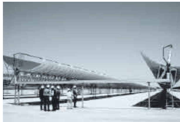
SKAL ET Parabolic Trough Collector loop, built by Solar Millennium AG and FlagSol into the operating SEGS V plant at Kramer Jct., California.
